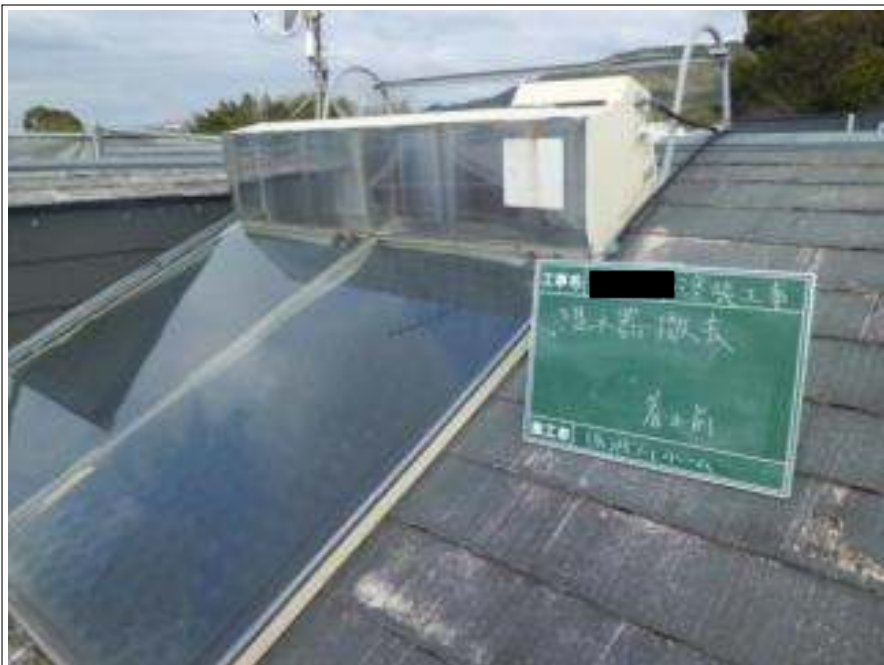
温水器撤去施工前
