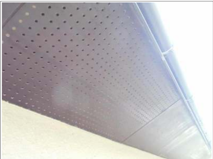
軒天塗装施工前
